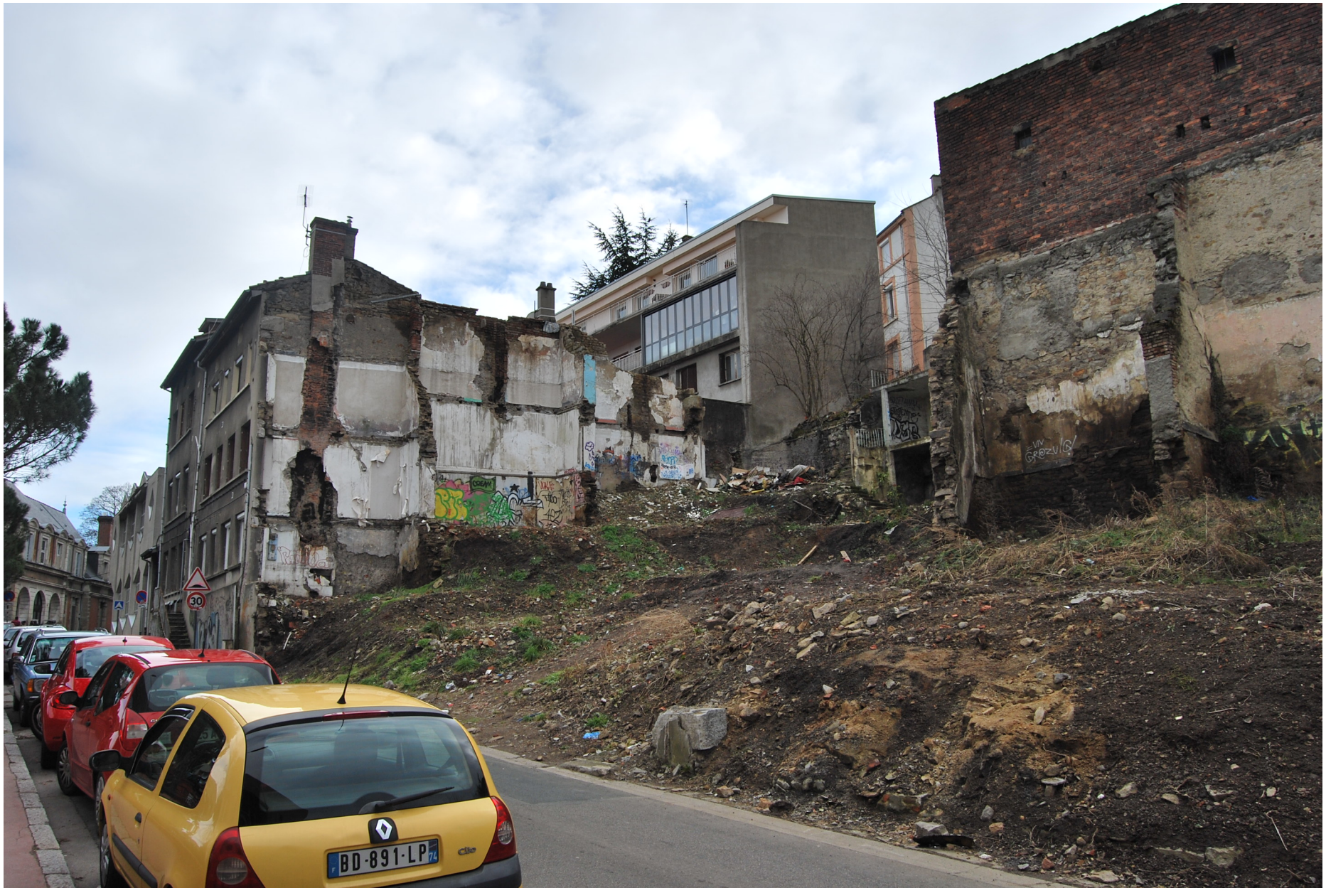
Demolition in Saint-Etienne
