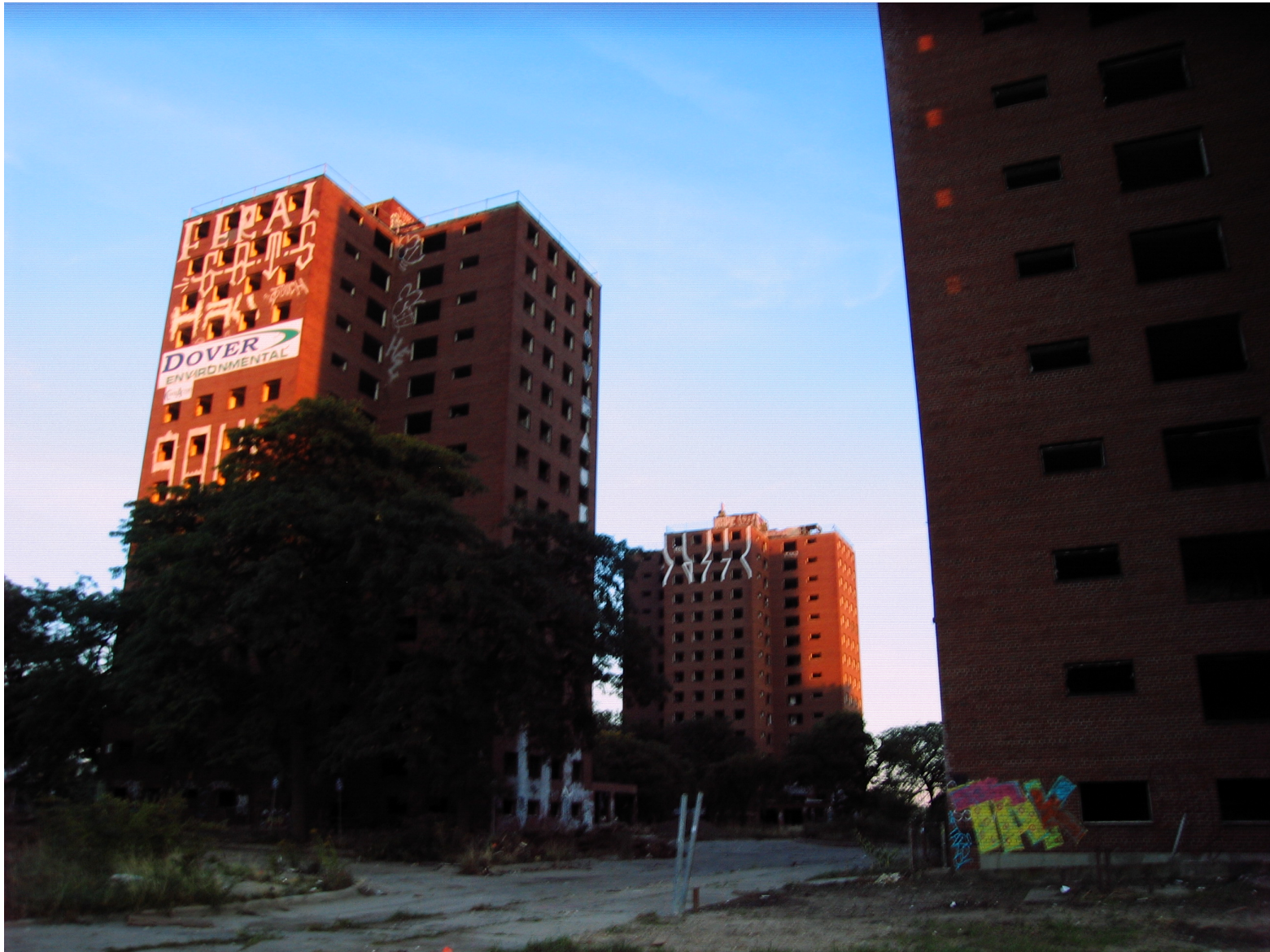
Demolition of social housing (Detroit)
