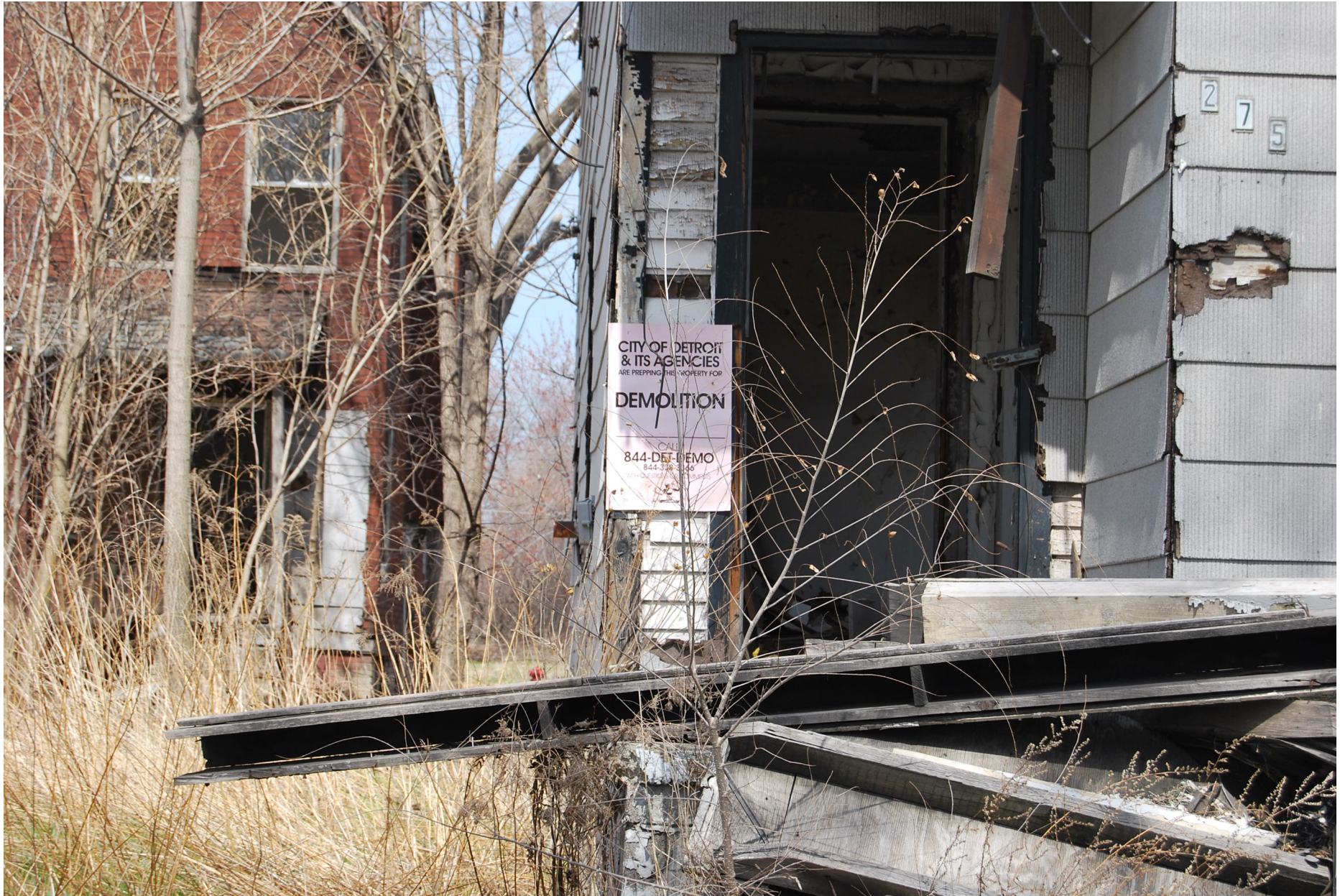
Demolition of private houses (Detroit)
